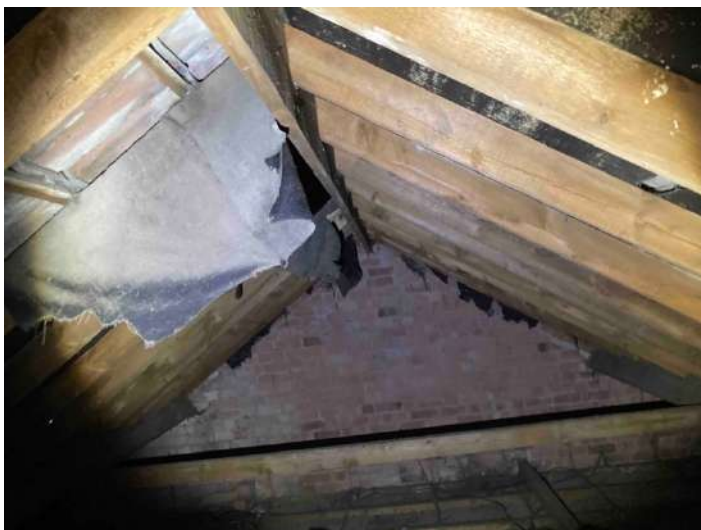
Image 7 – North end of roof void
