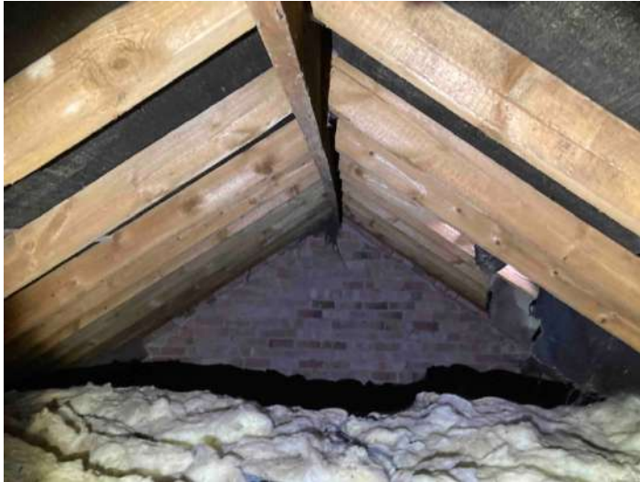
Image 5 – South end of roof void
