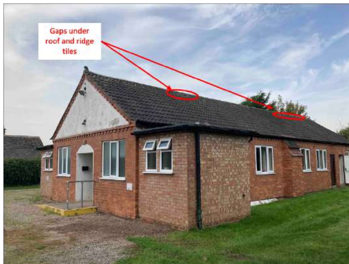
Image 2 – South and east elevations
