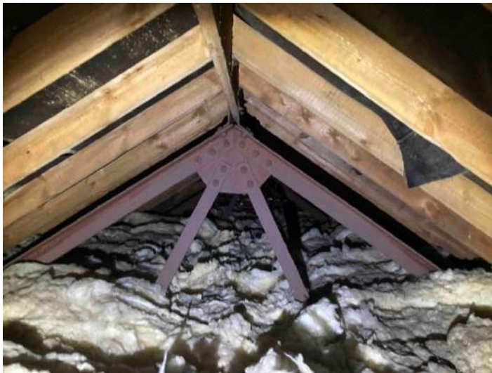
Image 6 – Central area of roof void
